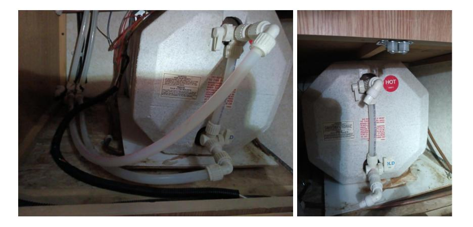
Remove the tank by pulling it from outside the coach. If it's too difficult, break away the Styrofoam from the HW tank for easier removal.
